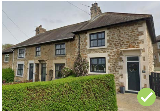
Figure 67: Materials and colour palette reflect the character of the Consett NA. The presence of detailing such as quoins and lintels elevates the quality of the building.
