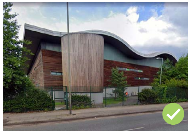
Figure 119: Gillmoss Recycling Centre, industrial can be architectural!
