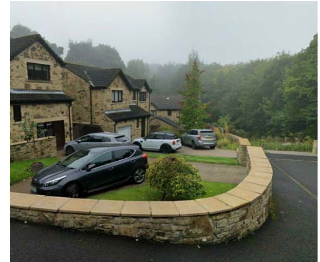
Figure 46: Stone rubble boundary walls have been used successfully at Goodwood Close. They reflect local character and respond to facade materials.
