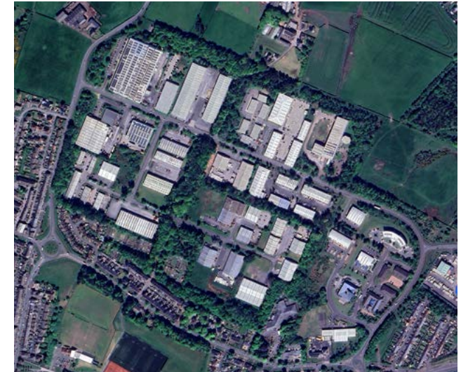
Figure 10: Number One Industrial Estate. Some distinct plots for development within the estate.
