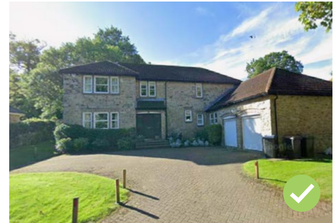
Figure 84: Good precedent of a detached house reflecting the character of Consett NA through the use of traditional colour tones and materials.
