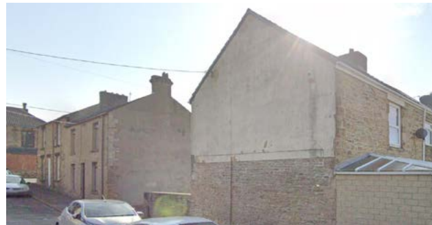
Figure 27: On side returns, where visible but not open to the street these may be rendered in one colour to match the rubble stone work.
