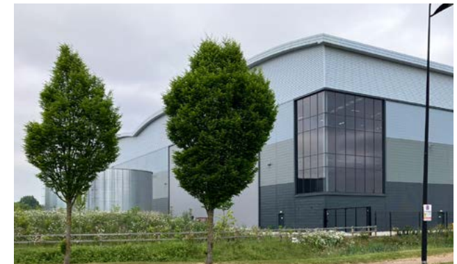
Figure 123: Muted tones and tonal variation (with darker shades at the base and lighter ones above), can help soften the silhouette of large buildings. Calder Park, Wakefield.
