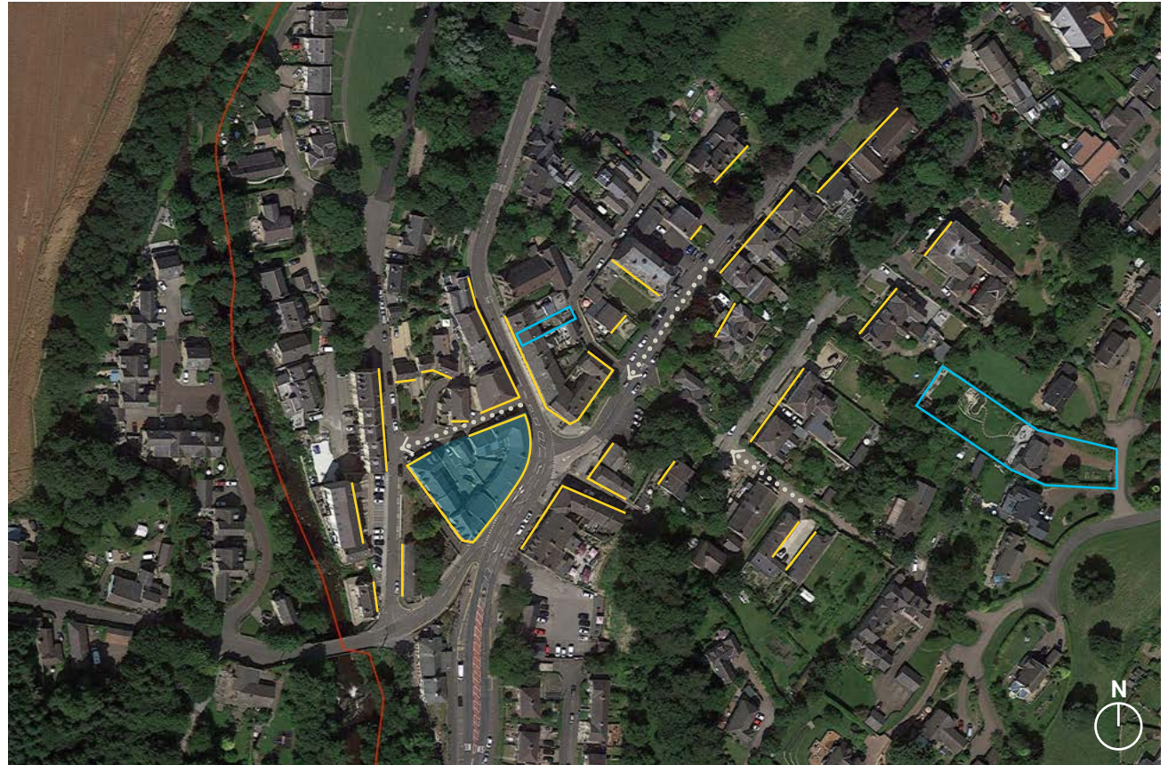
Figure 51: An aerial view of Shotley Bridge, one of the Historic Villages of the Consett NA.
