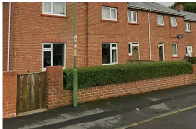
Figure 73: Neat brick wall and hedge Rutland Road Moorside.
