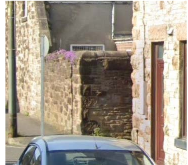
Figure 31: Rear boundary: rubble stone wall.
