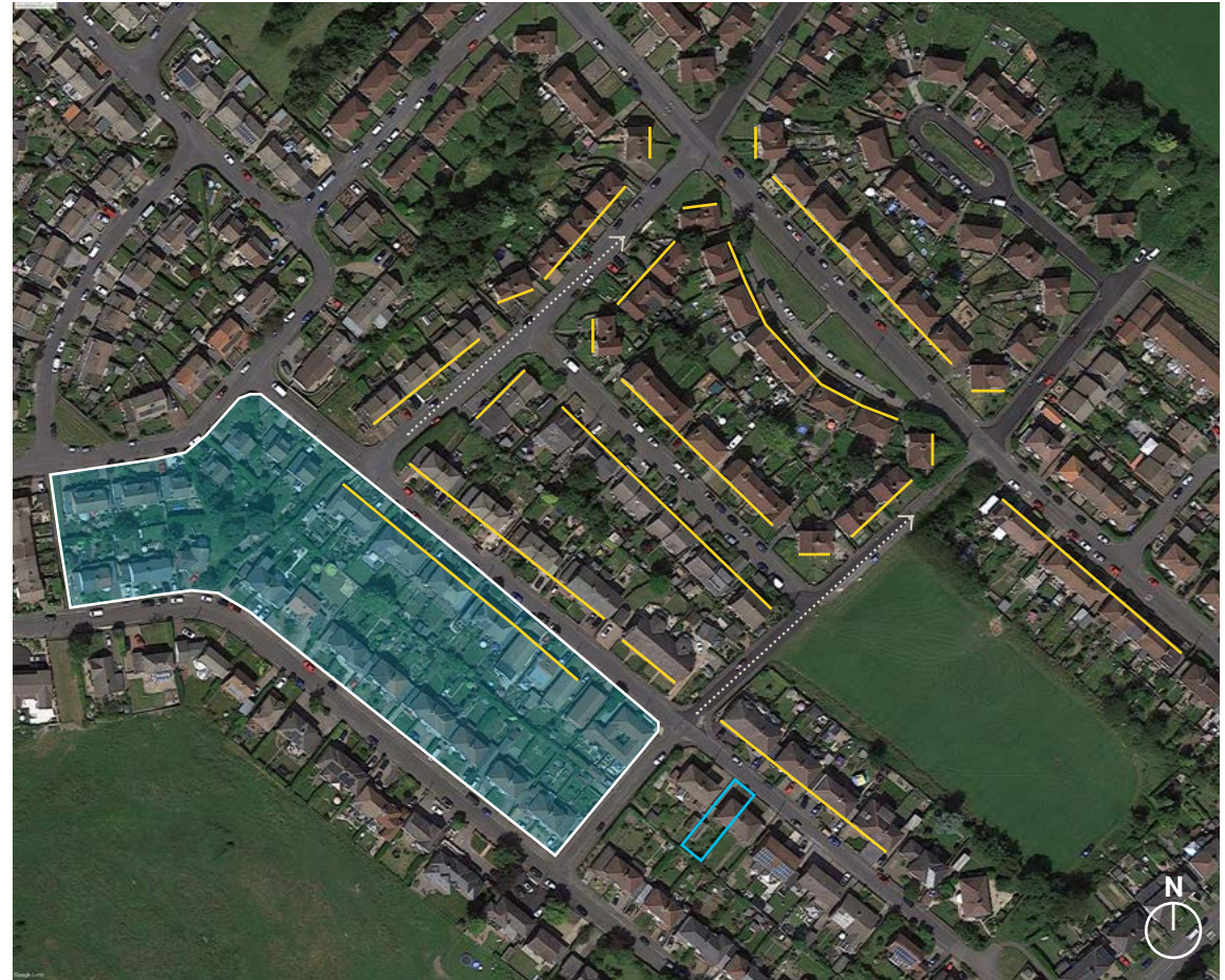
Figure 64: An aerial view of 20th Century suburban development in Bridgehill.
