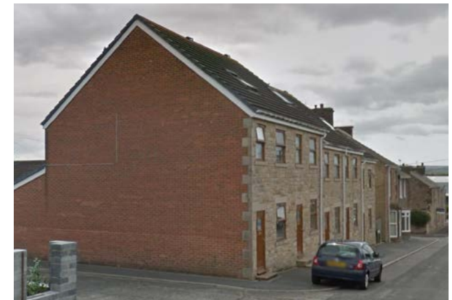
Figure 24: Modern example of terraced housing with street-facing facades make an effort to mirror traditional form, however the large brick gable spoils the visual elusion. Blank facades and large contrasting areas (material/colour) should be avoided.
