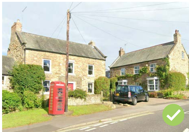
Figure 54: Variation in building orientation (with some frontages facing the street, and some rotated by 90 degrees) creates an interesting streetscene.
