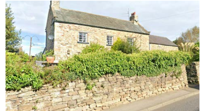
Figure 60: Traditional boundary treatments include dry stone walls, often in combination with planting.
