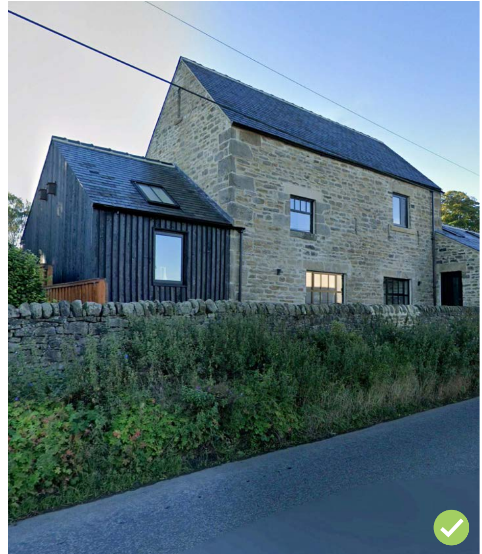
Figure 63: An innovative home extension in Ebchester, which makes use of contrasting (yet complementary) materials to mark it as different from the original structure. The extension is also subservient in form.
