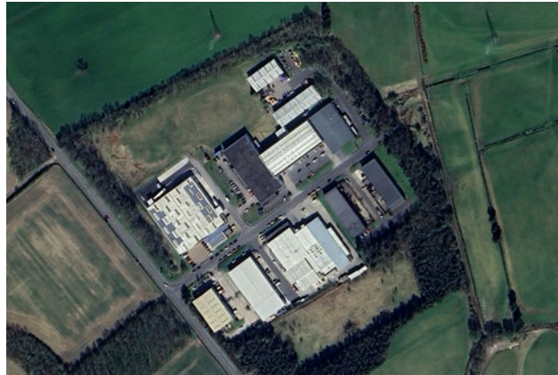
Figure 13: Leadgate industrial estate, small plot.
