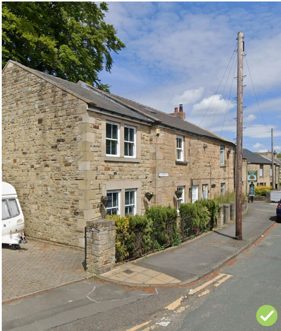
Figure 61: A sympathetic residential extension in Medomsley, which respects the existing form of the building and draws upon characteristic proportions and architectural features.
