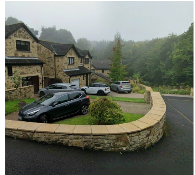
Figure 48: Stone rubble boundary walls have been used successfully at Goodwood Close. They reflect local character and respond to facade materials.
