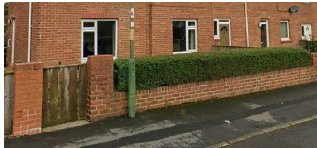
Figure 72: Neat brick wall and hedge Rutland Road Moorside.
