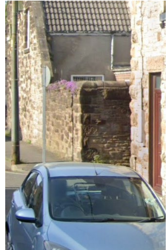
Figure 33: Rear boundary: rubble stone wall.
