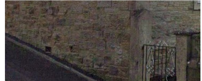
Figure 30: Rubble Stone to all elevations fronting the street. Use of quoins only on key junctions (cross roads). Random coursing.
