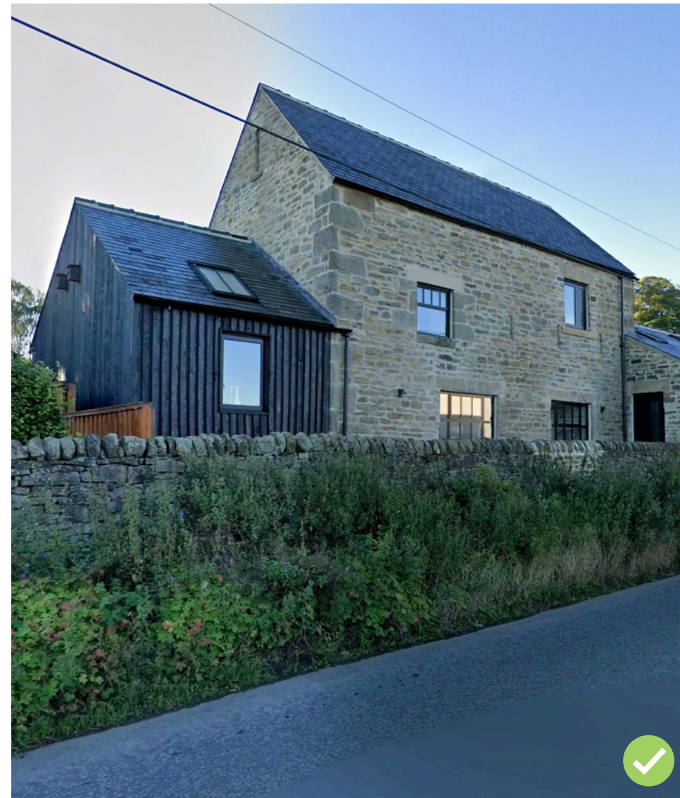
Figure 62: An innovative residential extension in Ebchester, which makes use of contrasting (yet complementary) materials to mark it as different from the original structure. The extension is also subservient in form.
