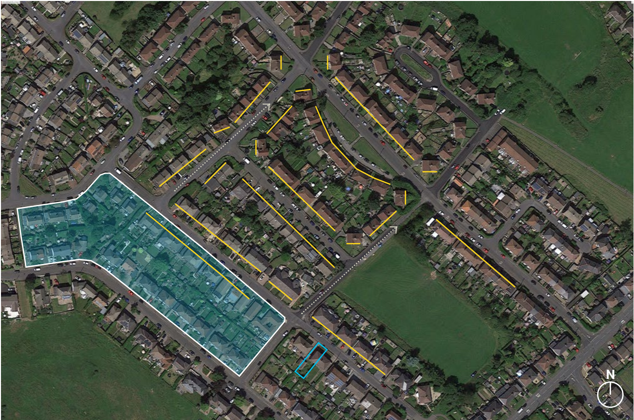
Figure 63: An aerial view of 20th Century suburban development in Bridgehill.
