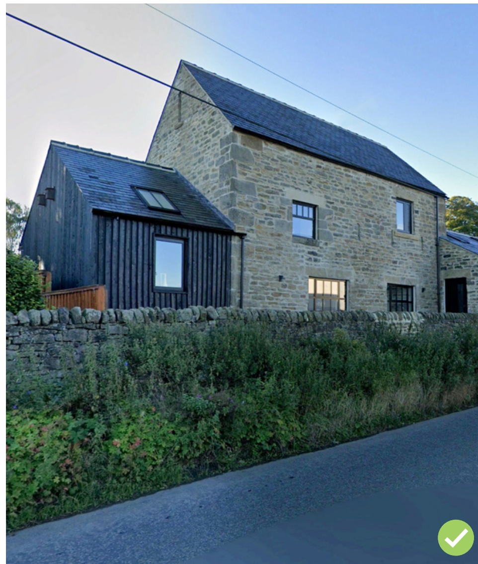
Figure 64: An innovative residential extension in Ebchester, which makes use of contrasting (yet complementary) materials to mark it as different from the original structure. The extension is also subservient in form.
