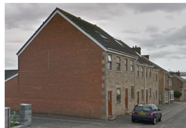
Figure 25: Modern example of terraced housing with street-facing facades make an effort to mirror traditional form, however the large brick gable spoils the visual elusion. Blank facades and large contrasting areas (material/colour) should be avoided.
